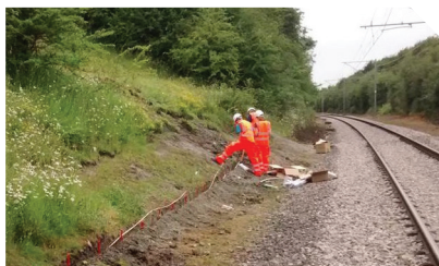
PRIME electrode installation
